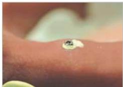
Cleaned surroundings of the pinhole
